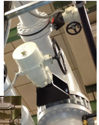
P7 Controlling Chiller Flow
