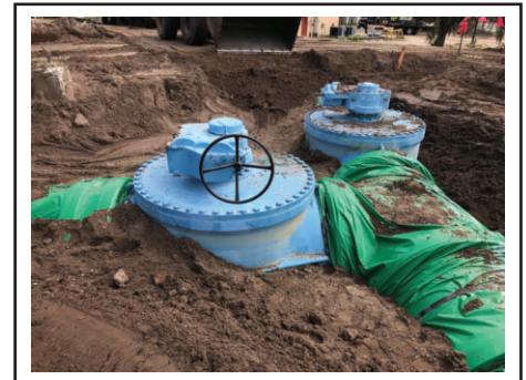
Cam-Centric® Plug Valve with worm gear actuator
