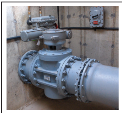
Cam-Centric® Plug Valve with motor actuator
