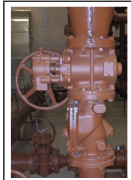
Cam-Centric® Plug Valve with Val-Matic Swing-Flex®
