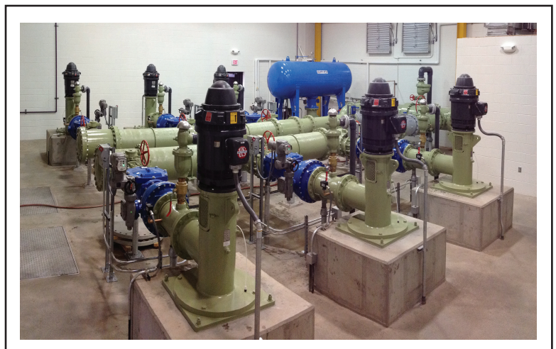
Air/Vacuum Valve with Dual Port Throttling Device for Vertical Turbine Pumps
