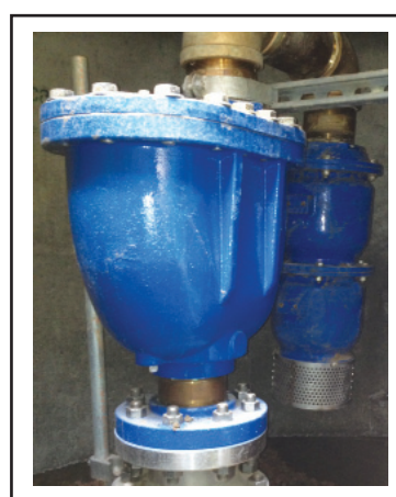
Single Body Combination Air Valve with FloodSafe® Inflow Preventer
