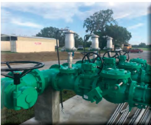
Cam-Centric® Plug Valves, Swing Check Valves & Combination Air Valves
