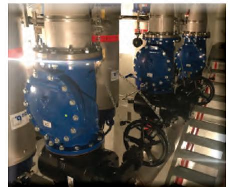
Swing-Flex® Check Valves & Cam-Centric® Plug Valves
