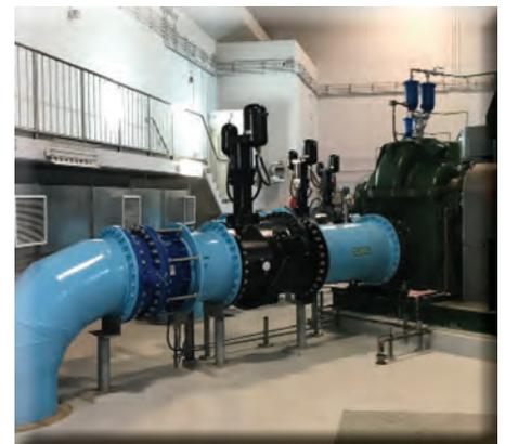
American-BFV® Butterfly Valves, Tilted Disc® Check Valves, Combination Air Valves & Silent Check Valves
