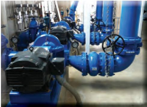
Air Valves, Silent Check Valve and American-BFV® Butterfly Valves
