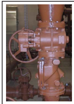
Cam-Centric® Plug Valve with Val-Matic Swing-Flex®
