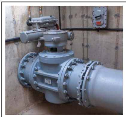
Cam-Centric® Plug Valve with motor actuator
