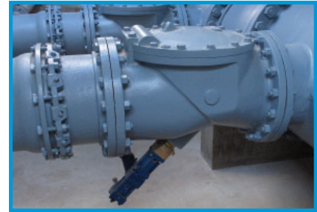
Swing-Flex® Check Valve with Oil Cushion for Pump Discharge
